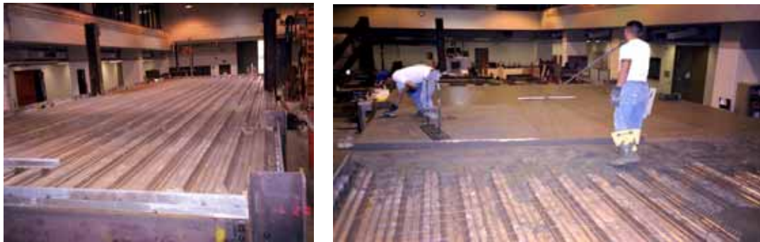
Figure 3.6. View of the specimen prior to and during placing concrete
