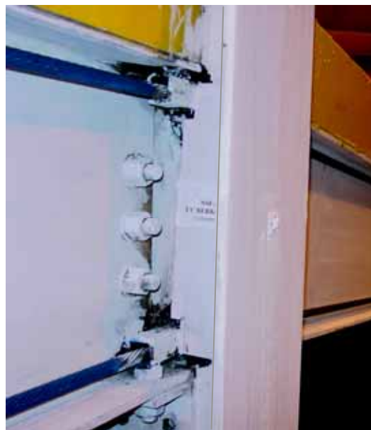
Figure 5.5. Cable Sleeves at Drop Column
