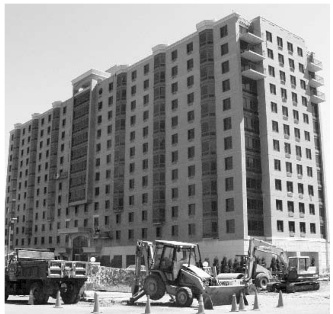
Fig. 1.3 Staggered truss apartment building.
